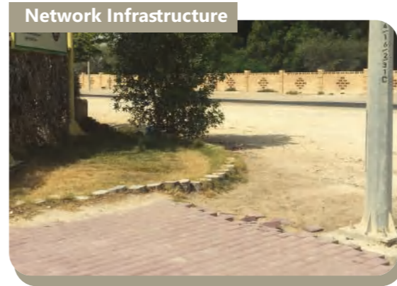
Discontinuous footway network and lack of connectivity.
